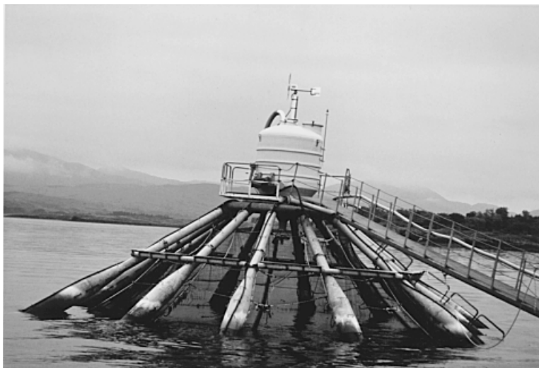
Fig. 6. A salmon net-pen in Scotland designed for use offshore, and in this case, exposed coastal waters.
