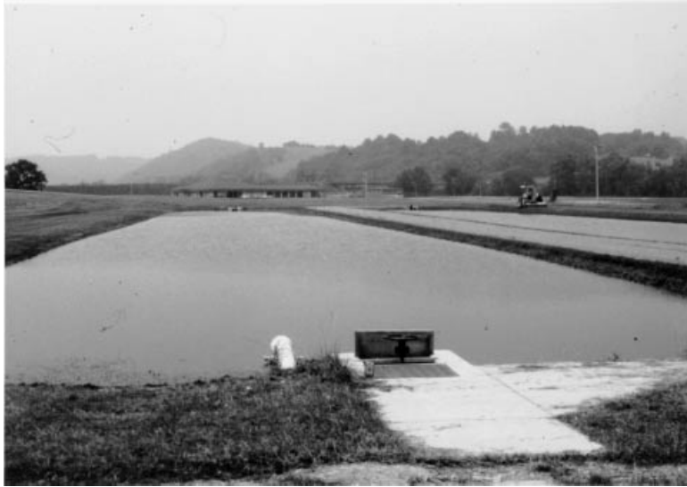
Fig. 2. Aquaculture ponds are often rectangular in shape. They should be equipped with plumbing for both inflow and drainage of water.
