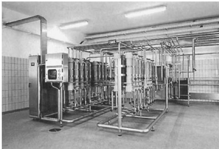
Fig. 3. A commercial dialysis facility showing the dialysis section of a German brewery where alcohol is removed from beer. Technical dialysis modules contain up to 50,000 capillaries and around 23 m 2 (250 ft 2 ) of membrane surface area. Typical plants might contain between 50 and 100 modules. (Courtesy of Holstein and Kappert Prozesstechnik GmbH, Dortmund, Germany.)
