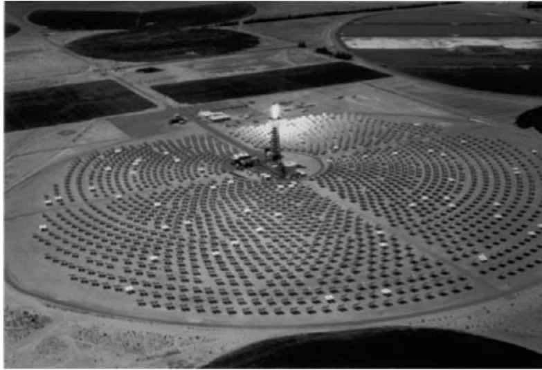
Fig. 3. The 10-MW Solar One plant, which advanced solar thermal power through the use of tracking mirrors to concentrate sunlight onto a central tower-mounted receiver.(Courtesy of Southern California Edison.)
