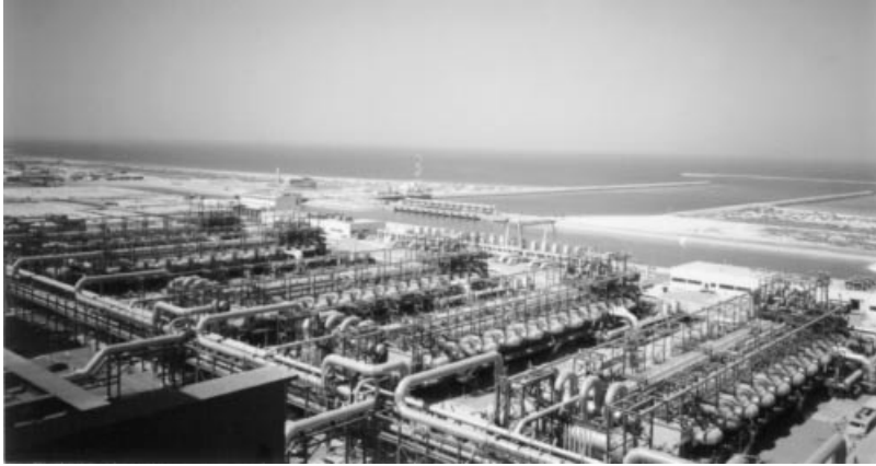
Fig. 4. The 341,000-m 3 /d multistage flash (MSF) evaporation desalination plant Al Taweelah B in Abu Dhabi, United Arab Emirates. Courtesy of Italimpianti SpA. It is a dual-purpose plant, composed of six identical power and desalination units. The desalination units at 56,800 m 3 /d each are currently the largest in the world. They have 17 recovery and 3 reject stages and a Performance Ratio of 8:1. The plant also produces 732 MWe of power.
