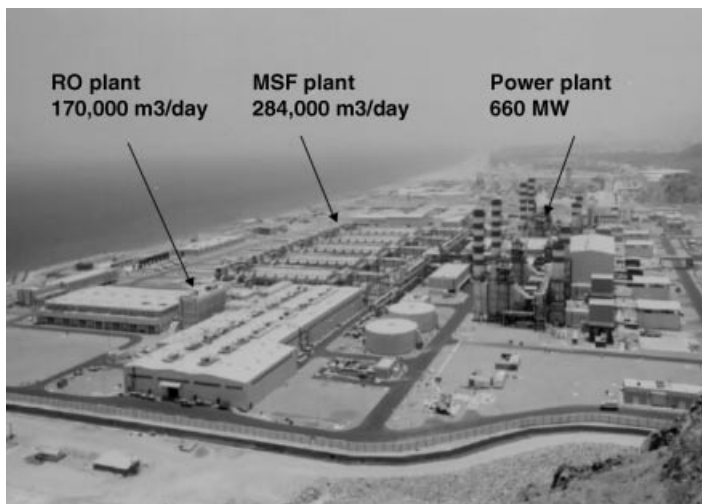
Fig. 27. Fujairah hybrid desalination complex, net output: power 500 MW, water 454,000 m 3 /day. (Courtesy Doosan Engineering.)
