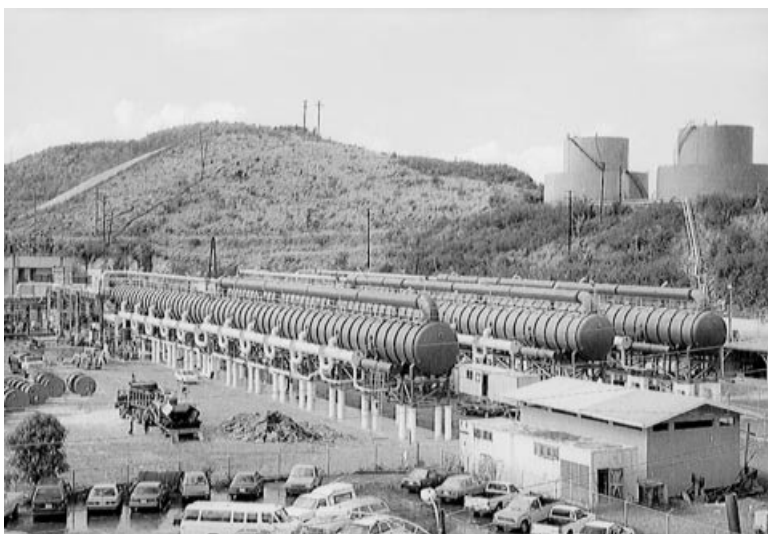
Fig. 5. A horizontal-tube multi-effect (HTME) desalination unit, producing 5000 \text{m}^3/\text{d} in St. Croix, U.S. Virgin Islands. Courtesy of I.D.E. Technologies Ltd.
